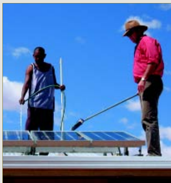
Maintaining Bushlight solar panels
